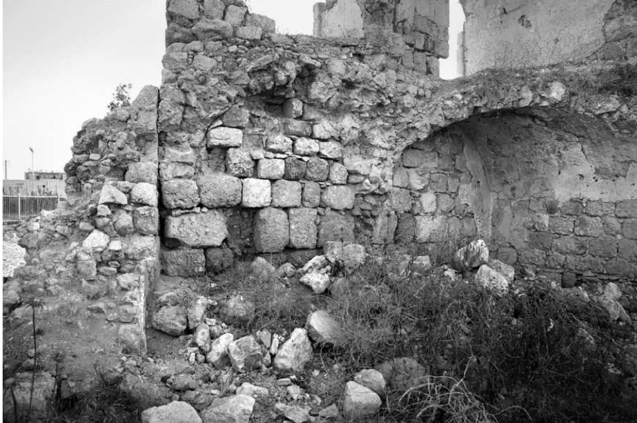
Fig. 3. The western enclosing wall and the walls of the southern wing built against it
